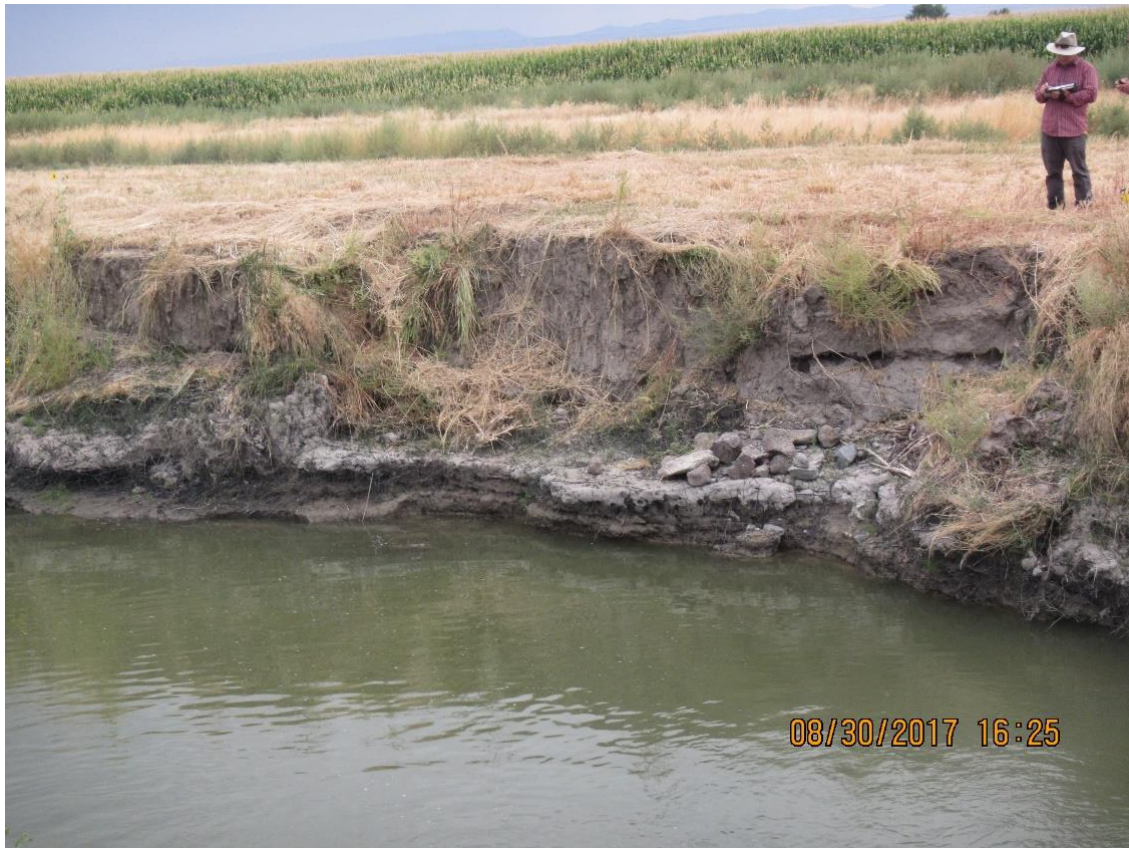
Figure 1-7. View of eroded right bank channel wall facing slightly downstream.
