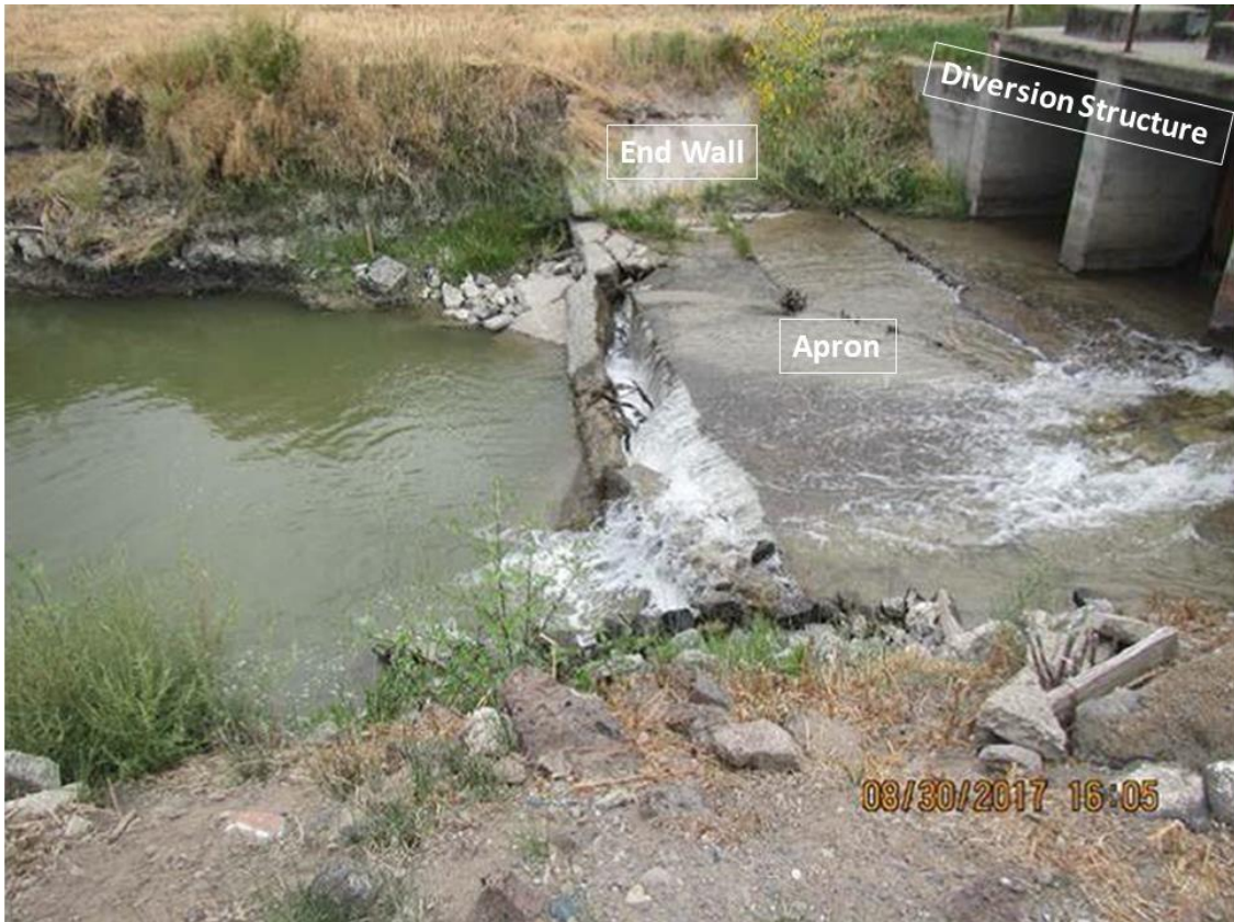
Figure 1-4. View of end wall of concrete outlet apron.
