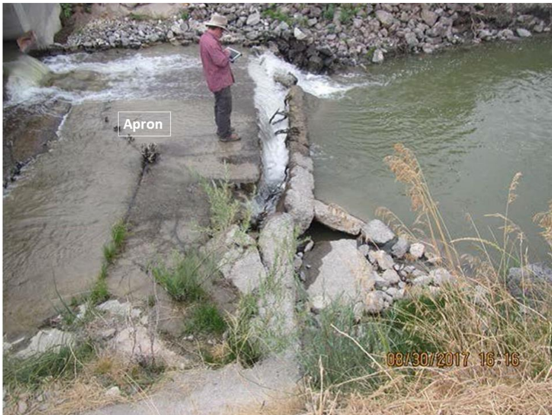
Figure 1-5. View of concrete outlet apron from right bank.
