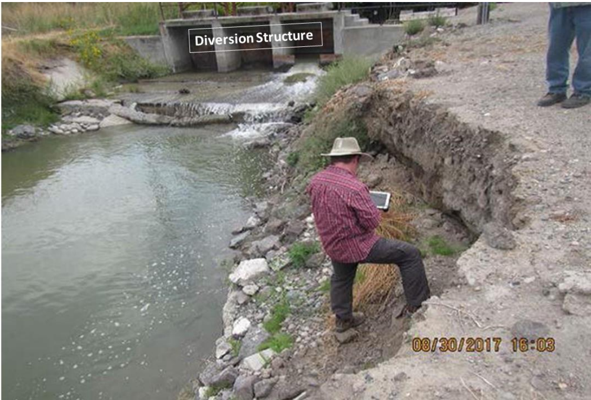
Figure 1-6. View of diversion structure and eroded left bank channel wall facing upstream.
